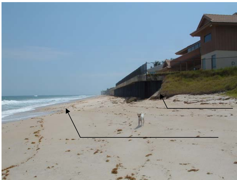
Figure 2 This house shows the dramatic difference between beaches with armament and the natural position of the beach.
