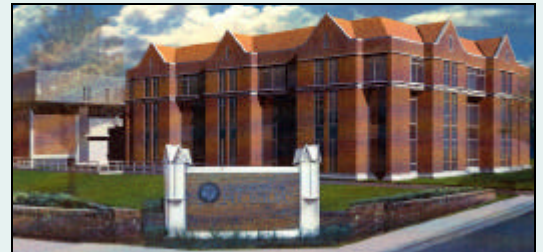
Work will begin soon on an expanded College of Law library and new Student/Faculty Center.
